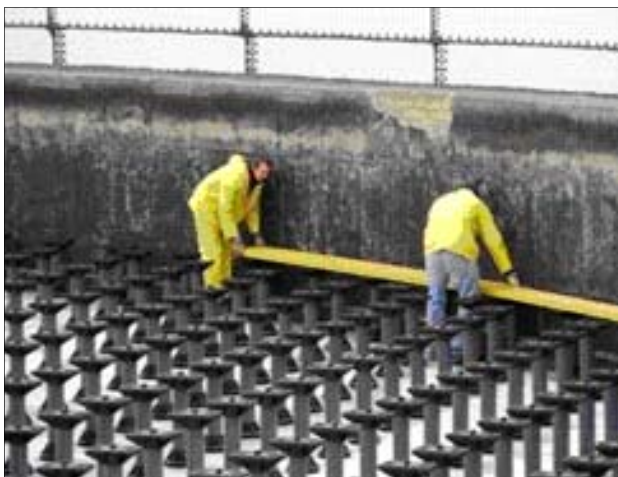
Owner Installation of Media Support System
